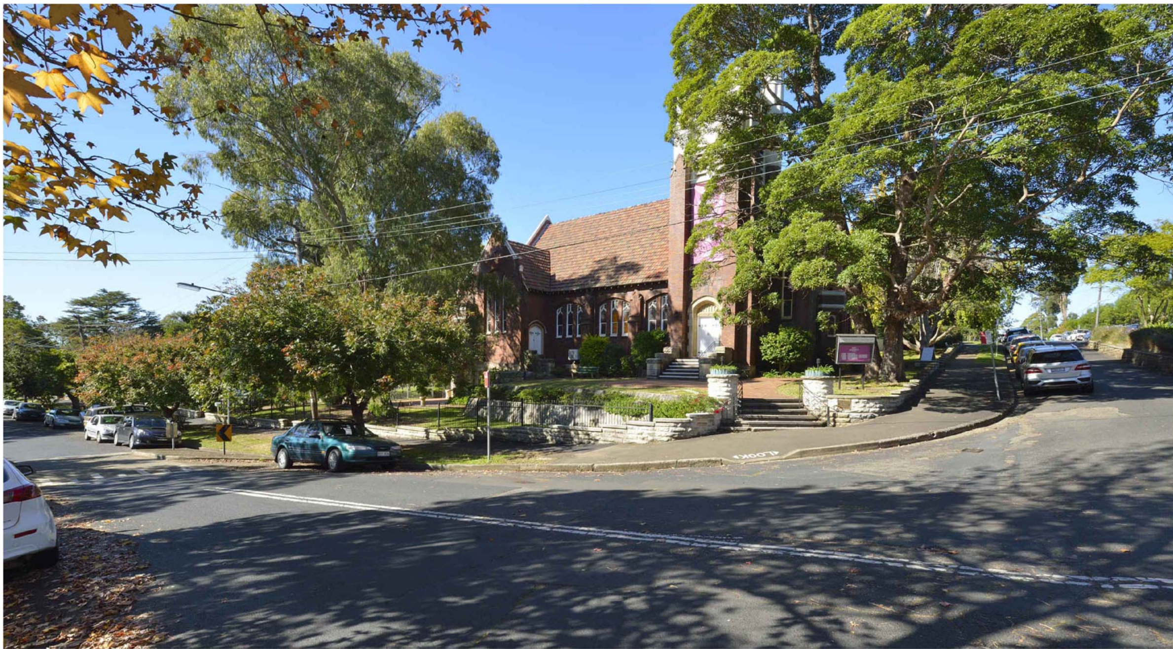
01 EXISTING BANCROFT AVE & HILL ST CORNER EXISTING STREET VIEW NTS
